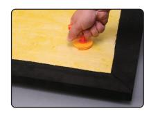
Screw the Snap-On Anchors into the back of the panel using the Snap-On Hex Driver tool. Making a small slit with a utility knife can aid in starting the anchors insertion.
