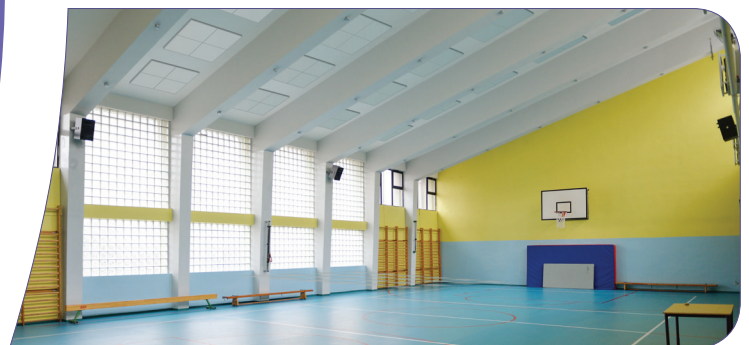
White SoniCell panels installed on ceiling
