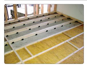
Any size flooring joists (must be 2" nominal – i.e.  $1\frac{1}{2}$ " wide to fit **U-Boats**<sup>TM</sup>) will work for walls or floors, but again, the larger the air cavity created by the joist, the better the potential decoupling effect.
