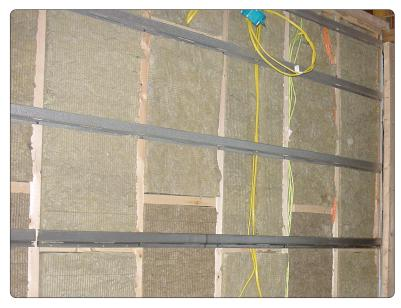
**RC-8's** are specially shaped metal to which gypsum board or other building materials can be mounted to isolate them from the framing members (studs) of a wall or ceiling. **RC-8 Resilient Channel** can add as much as 10 dB of isolation if used properly.
