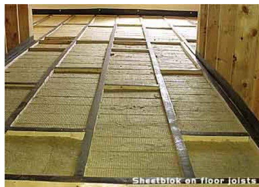
The right way to build a floor by following the Auralex system. Even if you can't build a new floor, though, there are effective steps you can take.
