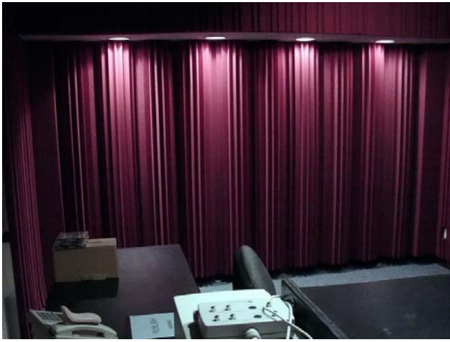
Sunburst Male Broadband Absorbers installed on the back wall of one of the Auralex studios. Consider doing this to a wall or your studio, iso room or iso booth for excellent low-frequency control.
