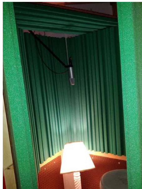
The corner freestanding, makeshift booth of Chris Vournazos, made of Auralex Metro on portable composite panels. Note the cloud above. Some people may need a stand-mounted bass trap in the corner, but the quality of Chris's audio is outstanding. (Follow the link to the left to hear his audio demos.)
