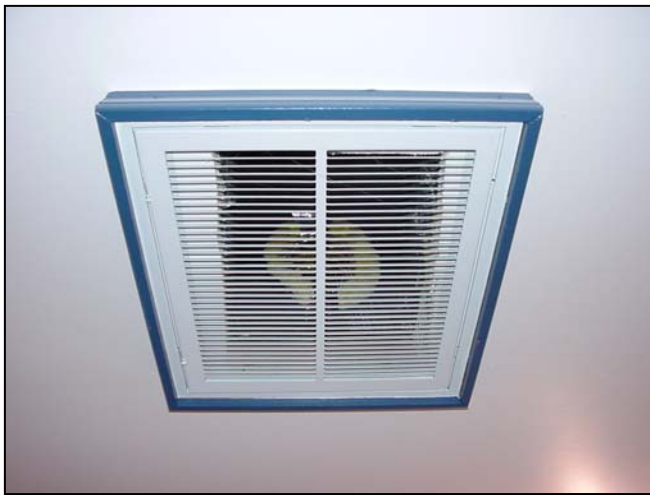
Figure 4.6a — Silent duct boot, grille closed
